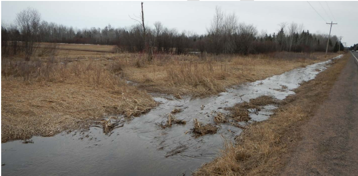
Figure 20. Ground view of roadside ditch conveying water during spring snow melt in April 2014. The shallow agricultural ditches shown in Figure 26 are seen in the upper left of this photo; they drain into this roadside ditch.
