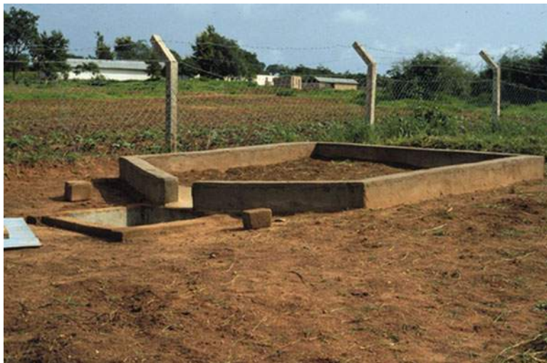
Fig. 3.19 A simple overland flow trap consisting of the contributing area delineated by concrete walls and a pit to collect water (Photo by Masaki Hayashi)
