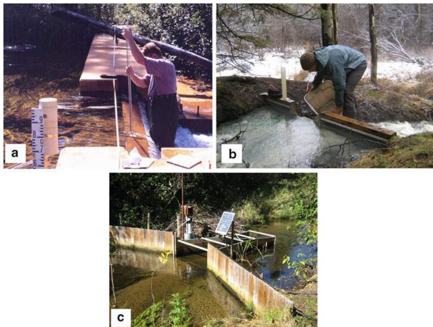
Fig. 3.11 Examples of artificial flow control structures: (a) a broad-crested weir in a stream in northern Manitoba, Canada, (b) a thin-plate weir in a stream in Banff, Canada, (c) a Parshall flume. The streamflow direction is from the left to the right in all photographs (Photos a and b by Masaki Hayashi; photo c by Donald Rosenberry)
