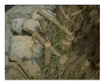
Bioengineering techniques are commonly used in stream restoration. Often they are combined with some measure of "hard engineering". Here poles have been set into bank. Below the poles rocks have been used to stabilize the bank.
