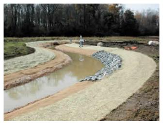
River and stream restoration projects involving both some "hard" and "soft" engineering including re-meandering and bioengineering are now common throughout the nation. This is stream restoration in Pennsylvania.
