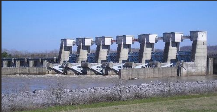
Old River Control Structure
