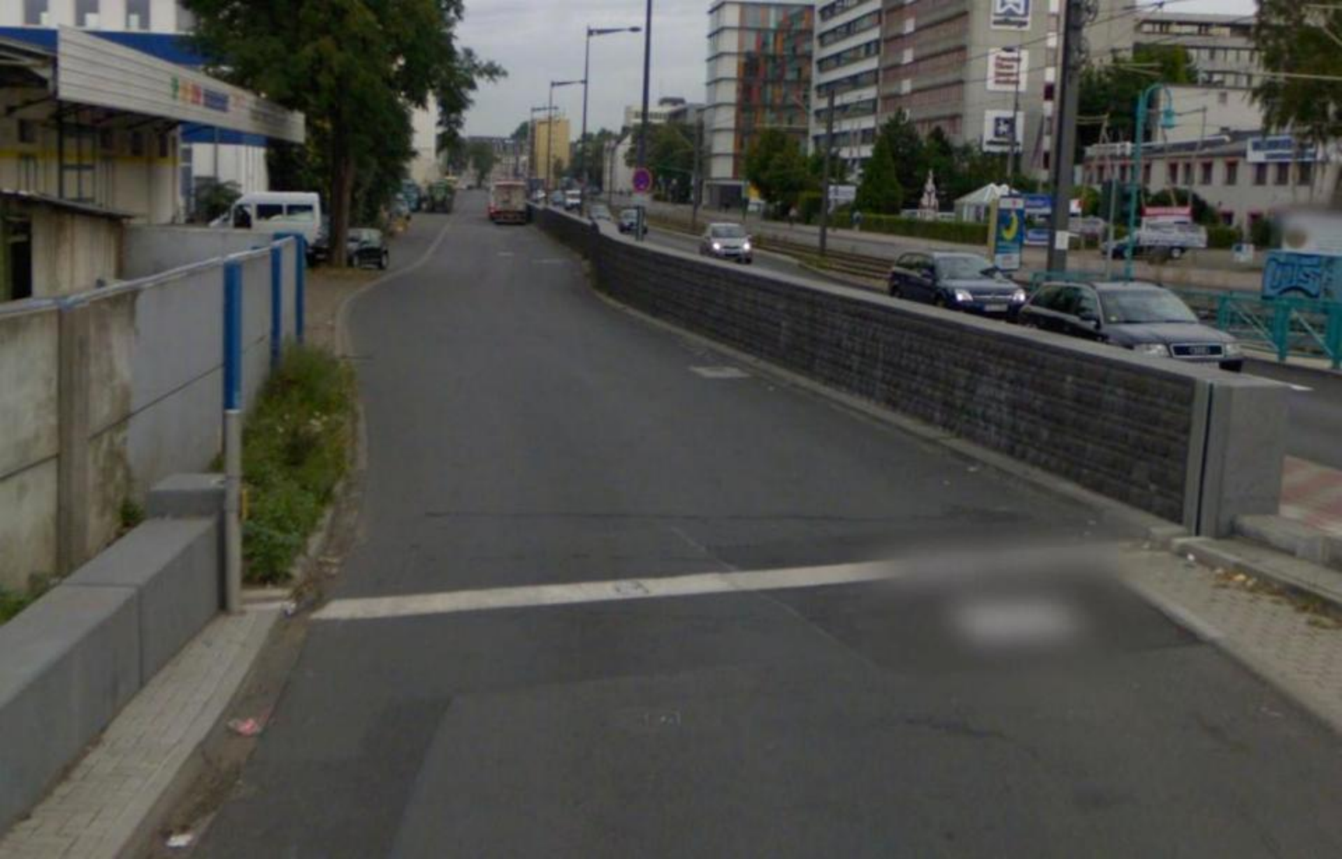
Floodwalls with removable aluminum or steel gates. Cologne, Germany (Rhine).
