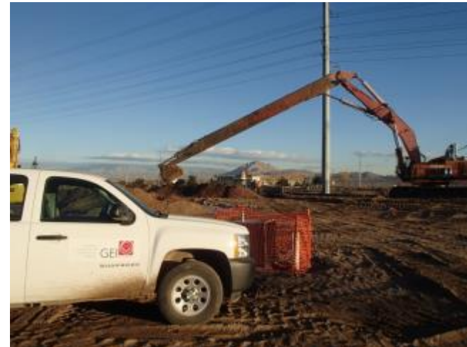
Soil Removal, Slurry Wall, GW Treatment, Landfills & Ponds - Nevada
