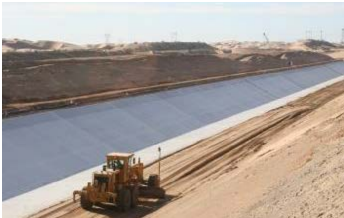
All-American Canal Lining Project Imperial County, California
