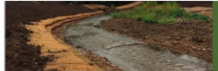
Soil lifts along Left Hand Creek following installation, but prior to planting and mowing.
