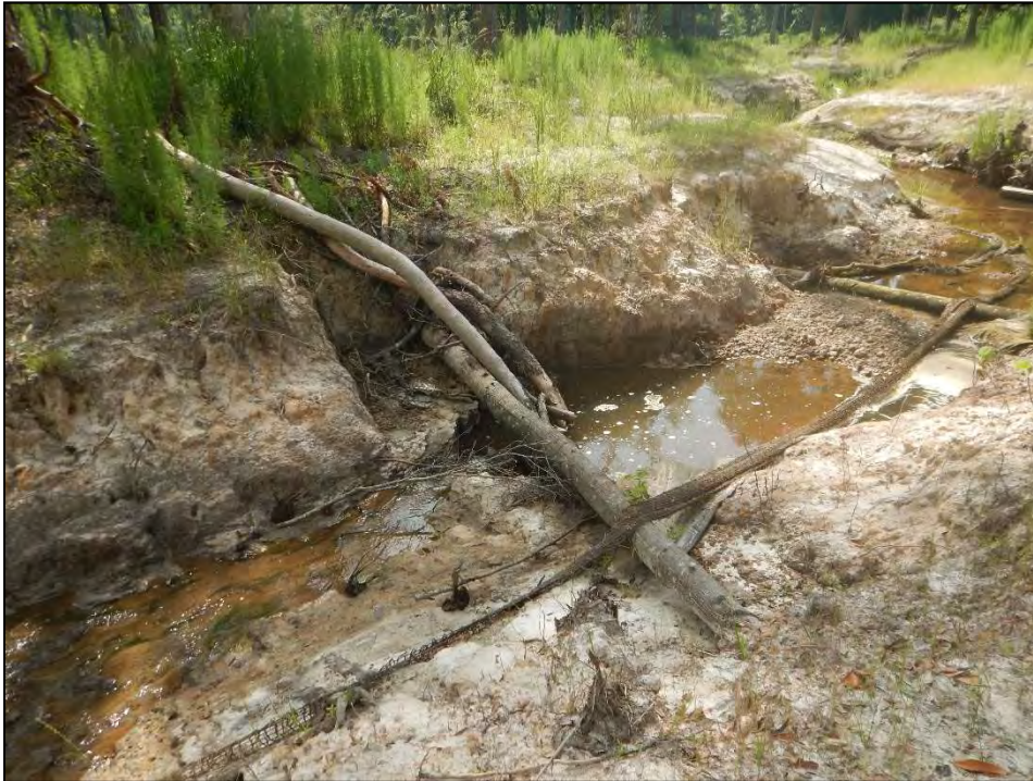
Channel Incision (Failed Grade Control Structure)
