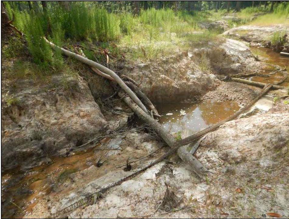
Channel Incision (Failed Grade Control Structure)
