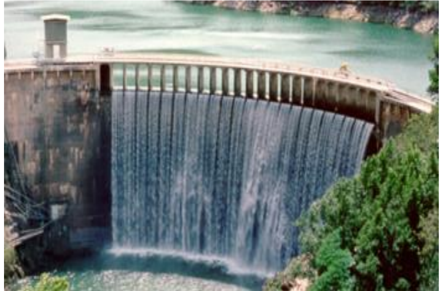
Former San Clemente Dam, Carmel River, California
