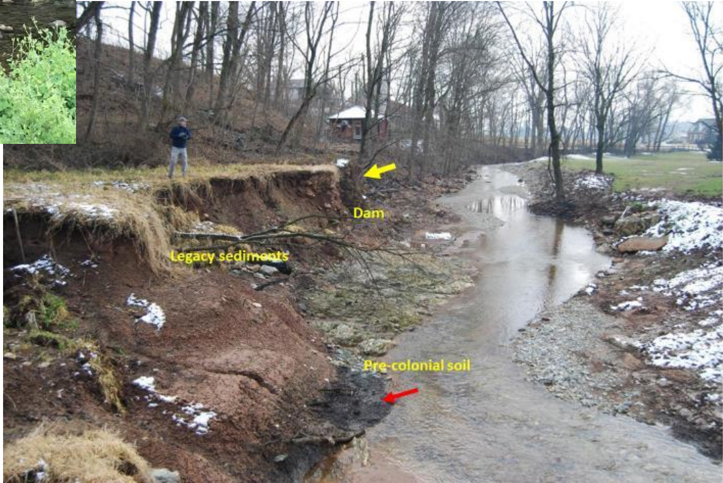
Stobers Dam Breach in 2011
