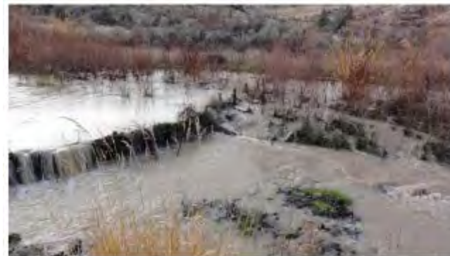
Figure 10. A typical stamper dam (SF-07 at Sanflower) with willow branches woven between vertical posts and the back side sealed with rock and clay. Note the dam height is sufficient to divert flow onto the RL terrace, mimicking a stable beaver dam.
