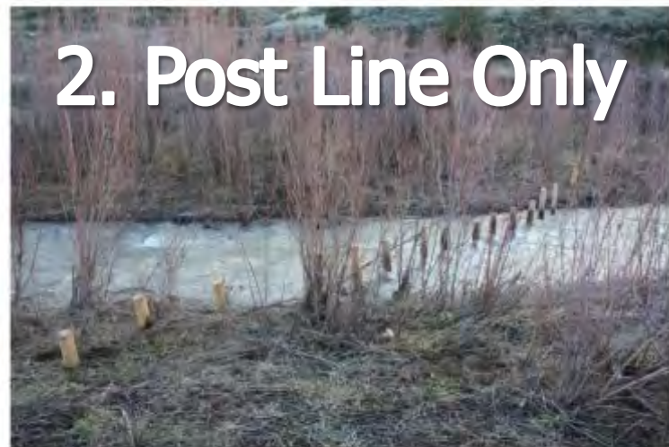
Figure 12. The purpose of a post line is to provide a site where beaver can build a stable dam. They generally create little or no geomorphic changes unless utilized by beaver.
