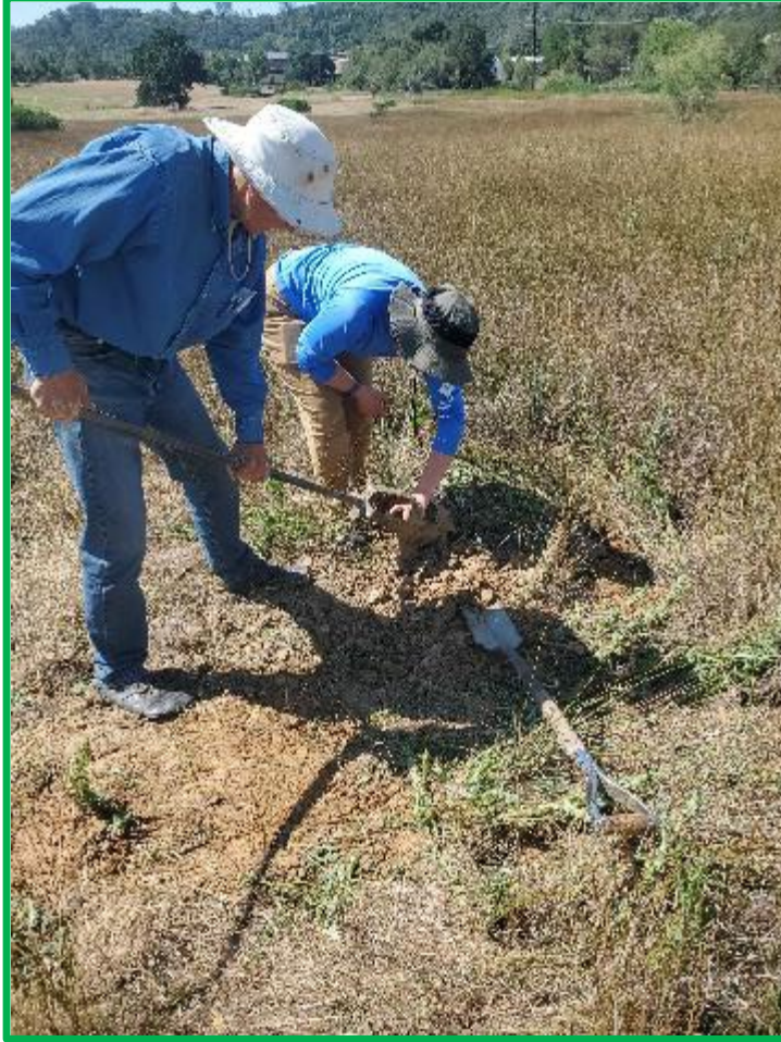
Installing the monitoring wells
