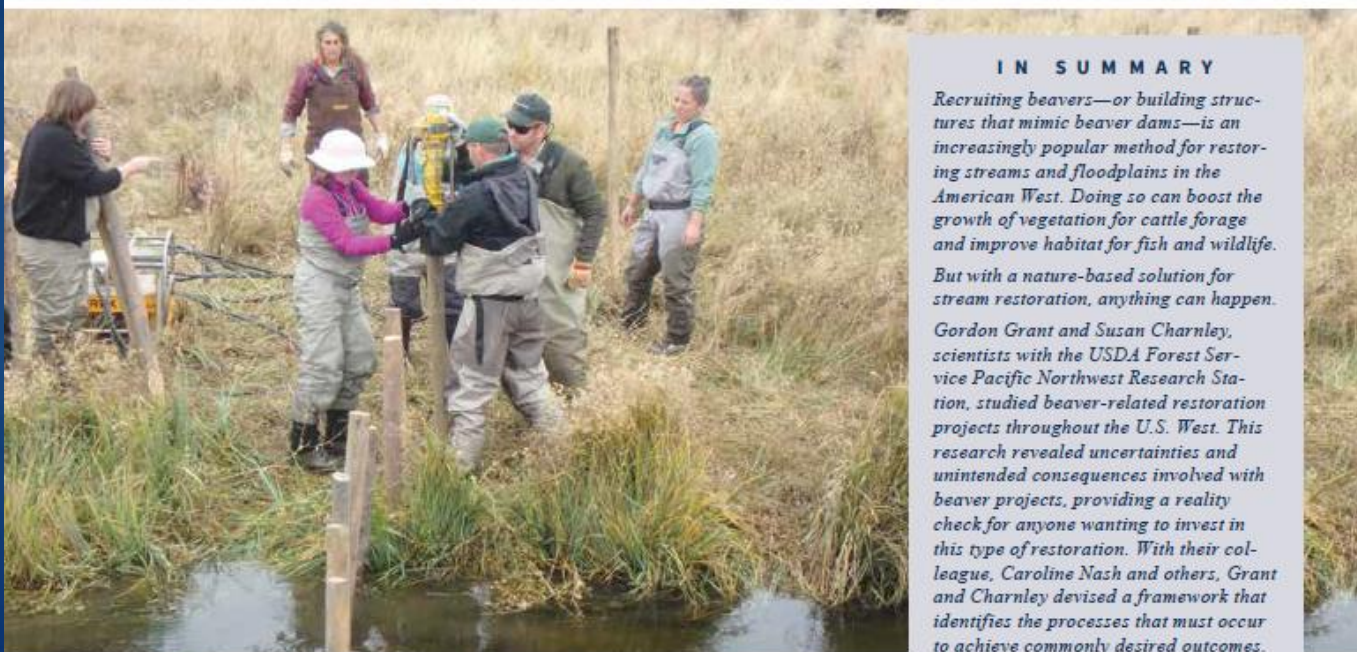
A work party builds a beaver dam analog in Bridge Creek, Oregon, a tributary of the John Day River. Beaver-related restoration tactics are being used to restore riparian areas, expand wildlife habitat, and improve forage for livestock. USDA Forest Service photo.
