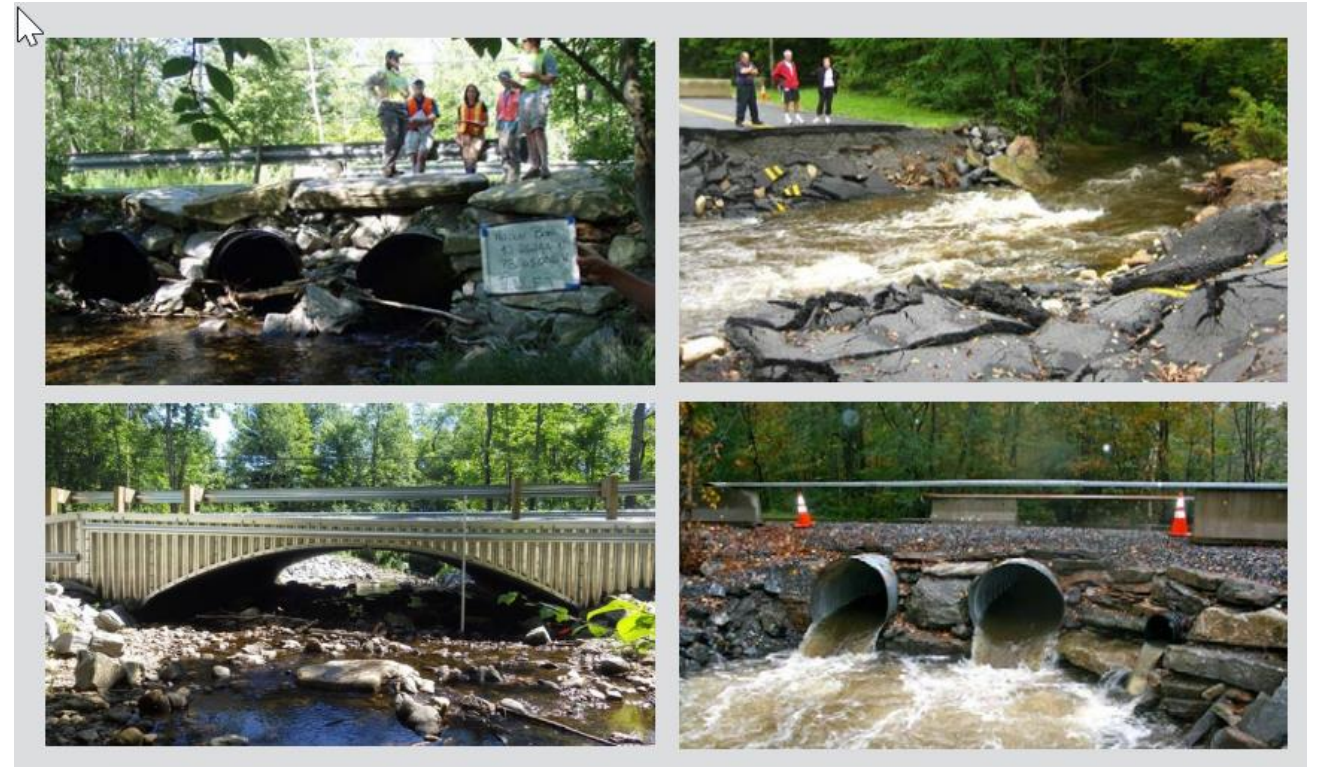
Clockwise from Top Left: 2009 (Pre-storm), 2011 (Post-hurricane Irene), 2011 (Temporary Replacement), 2016 (Replacement Bridge)
